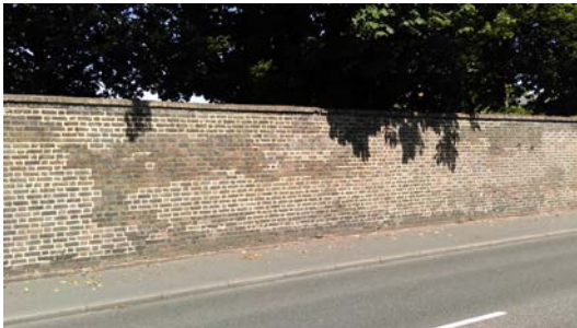
The brick wall forms part of the boundary to the Conservation Area
