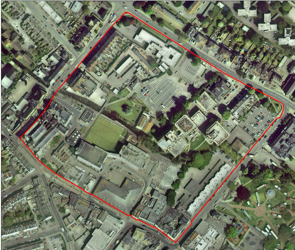
Aerial photograph of Mid Town
