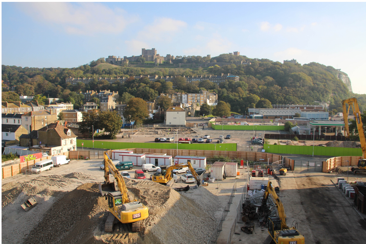
Figure 11.4 Elevated view of St James's site, illustrating the demolition works
