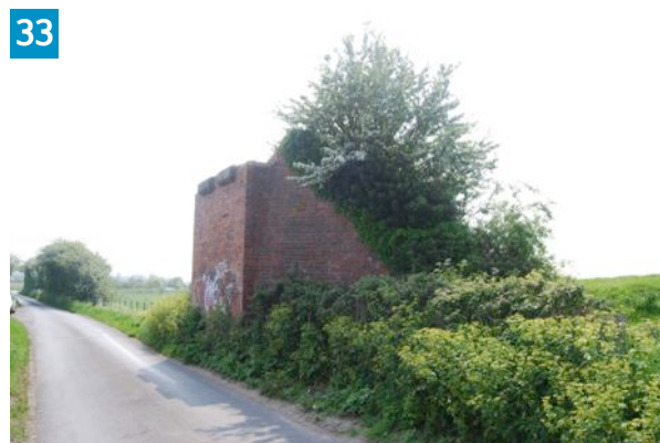
Figure 32 The remains of Sinker's huts found at Betteshanger Colliery during redevelopment of the site Figure 33 Abutment for the East Kent Light Railway crossing Richborough Road
