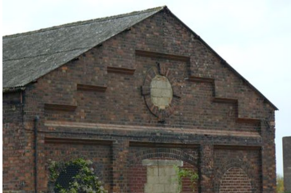
Figure 34 Architectural detailing on a colliery building at Snowdown
