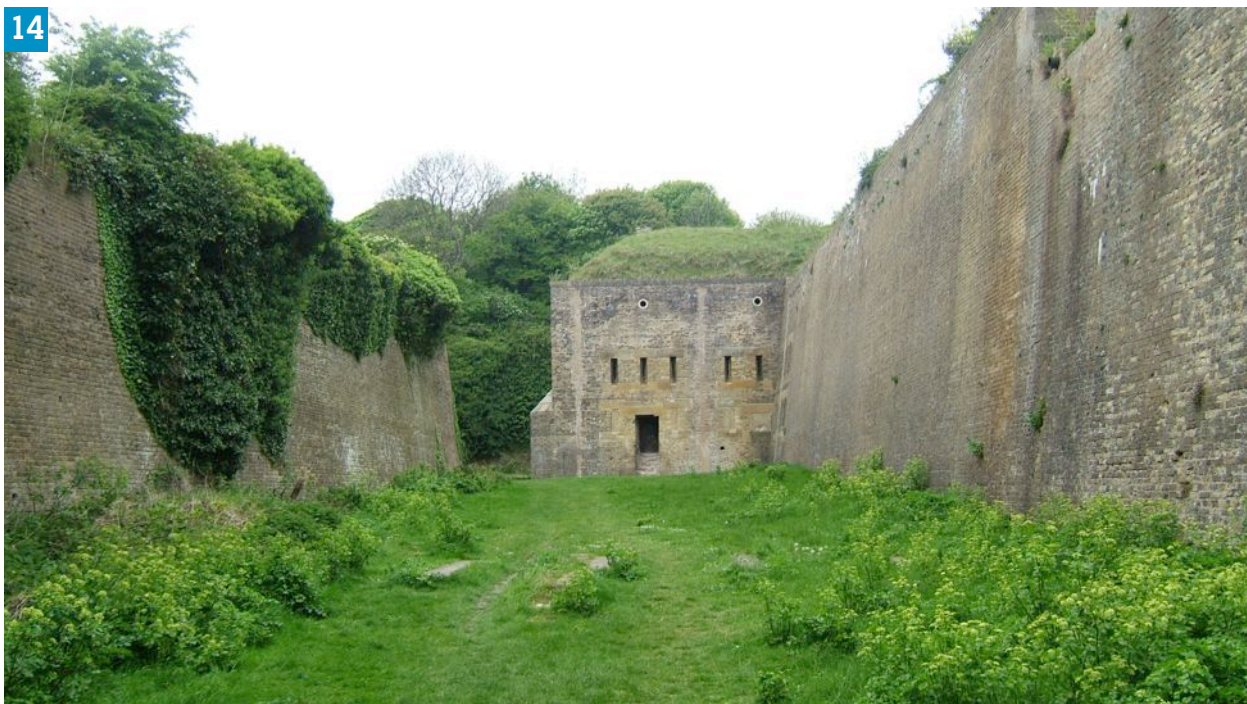
Figure 13 The Fairburn Crane in the Dover Western Docks is a Scheduled Monument Figure 14 The Western Heights
