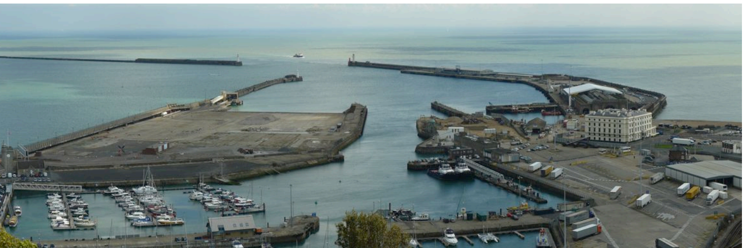
Figure 13 Dover Harbour, Admiralty Pier Extension battery and lighthouse Figure 14 Dover Harbour, Eastern Arm. © Dover Museum (d95583)
