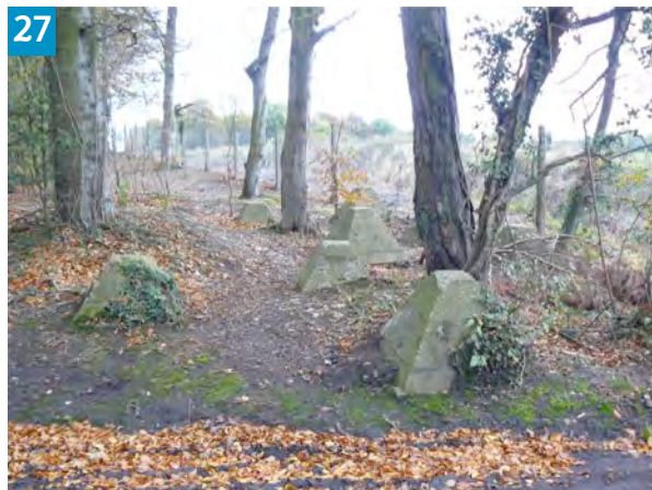
Figure 26 Scars for road blocks on a bridge over the Canterbury to Dover Railway Line
