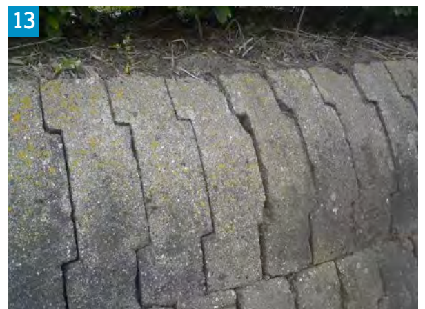
Figure 13 Prefabricated concrete sections for 'Moir' pillboxes originally cast at Richborough and intended for the Western Front. These sections were never used and now form a retaining wall near Woodnesborough
