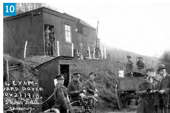
Figure 9 Partially exposed remains of the First World War period sound mirror at Fan Bay , east of Dover Figure 10 First World War checkpoint at Kearsney on the outskirts of Dover
