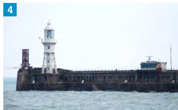
Figure 4 Pier extension battery at the western harbour entrance showing crew accommodation
