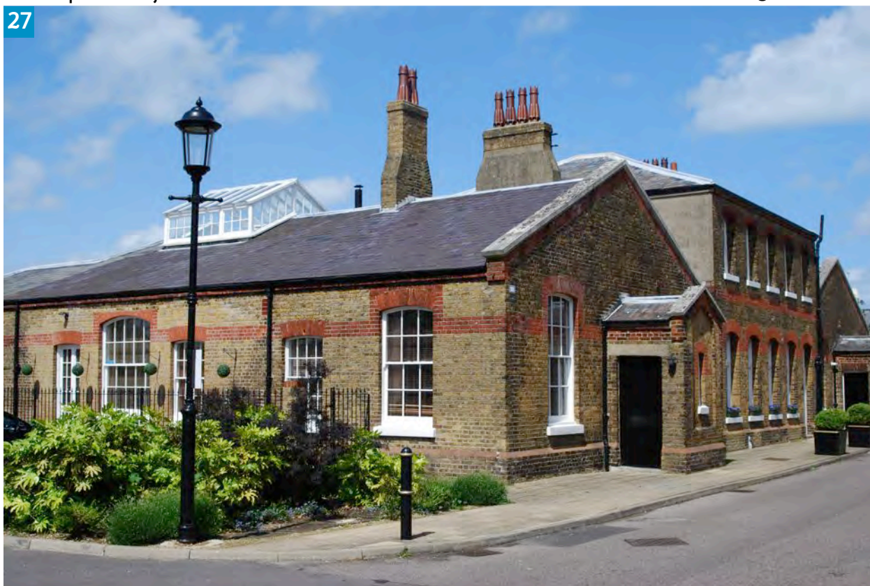
Figure 27 Former barracks buildings in Deal have been sympathetically converted to provide attractive residential properties
