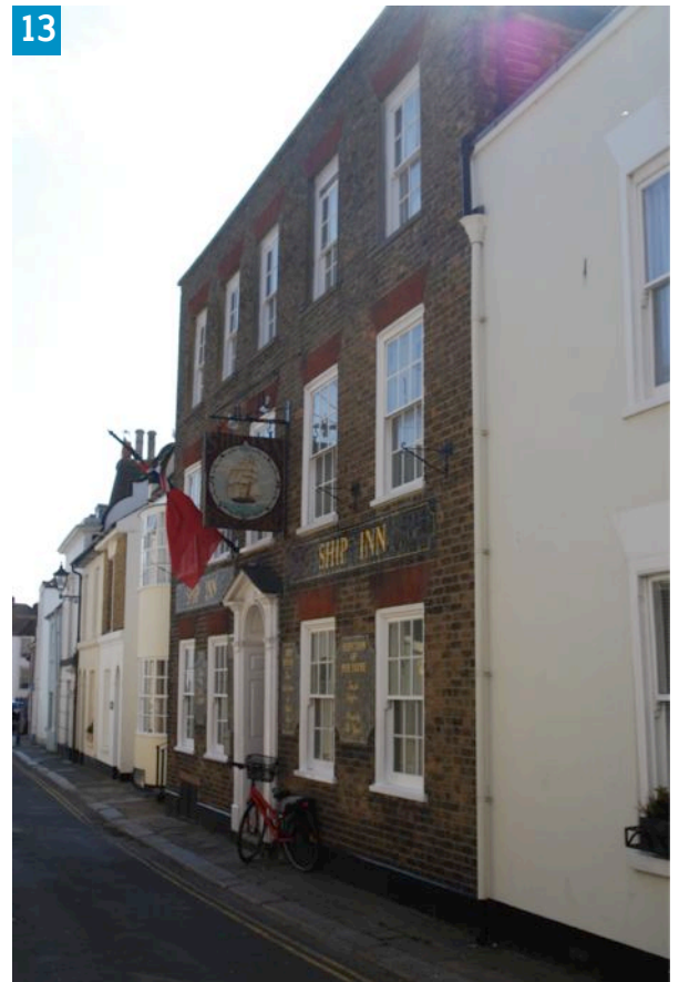
Figure 12 Port Richborough during the Great War. © Kent History & Library Centre Figure 13 The Ship Inn in Middle Street, Deal
