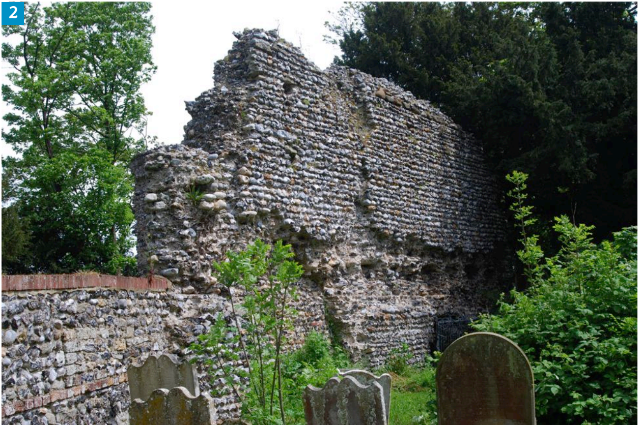
Figure 2 The ruins of Walmer Court, a fortified manor
