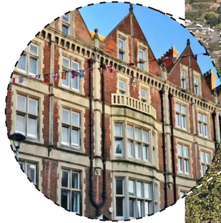
Red brick used on buildings along Cannon Street.
