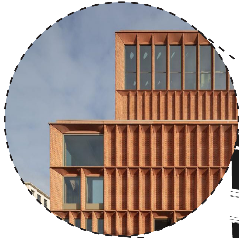
Full height glazing set within brick piers (The International Rugby Experience by Niall McLaughlin Architects)
