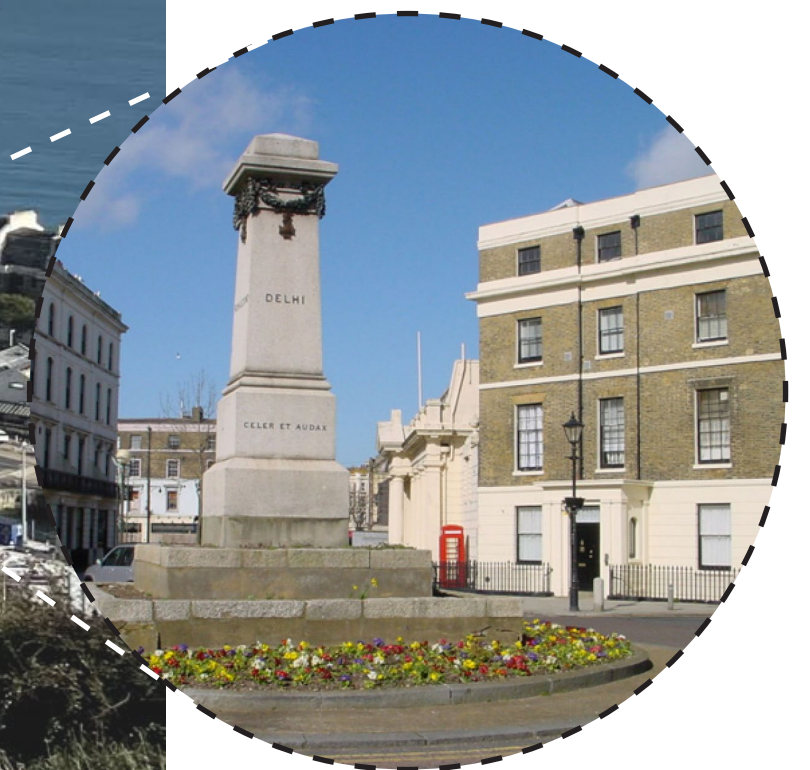
Stock brick used on buildings in Waterloo Crescent Conservation Area.
