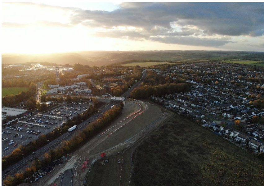
Image above shows 1b North (new bridge and embankment)
