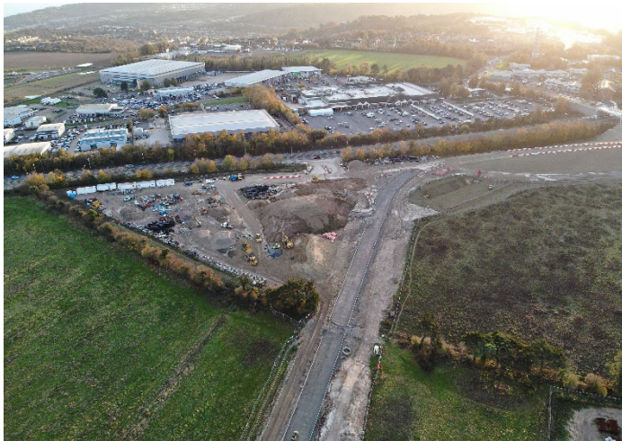
Image shows road construction in Section 1a/1b North prior to tarmac.
