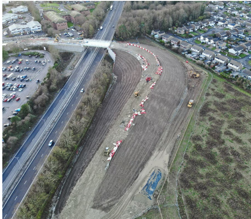
Image above shows 1b North (topsoil and preparation for tarmac)
