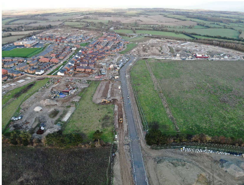
Image shows road construction in Section 1a/1b North prior to tarmac.
