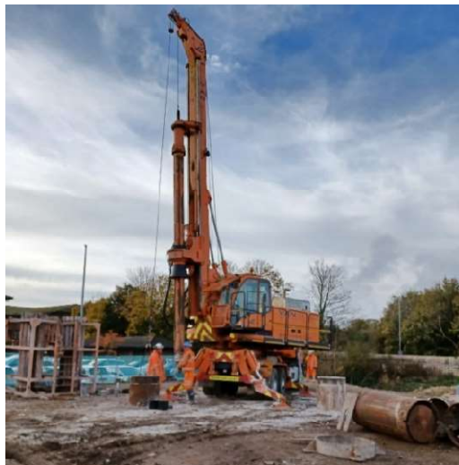
Installation of test pile cage and piling works
