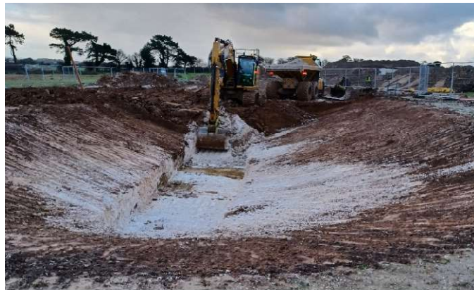
Digging out bio-retention pond
