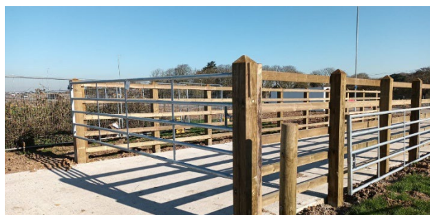
Timber post and rail fencing for Frith Farm cattle crossing
