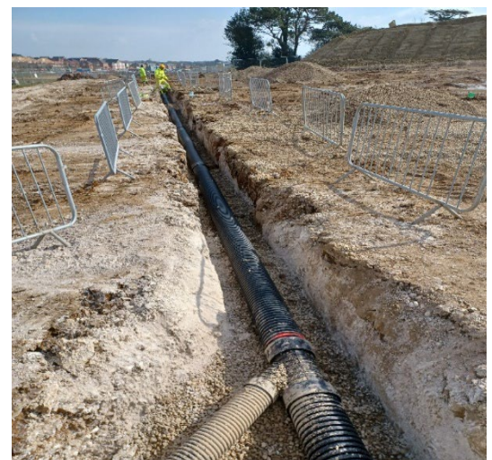
Installation of Drainage Pipes
