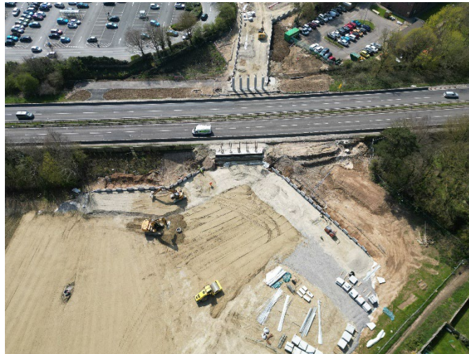
Drone photo of Section 1B North and South
