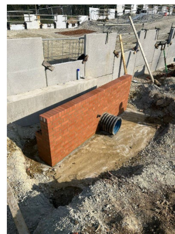
Completed brick headwall
