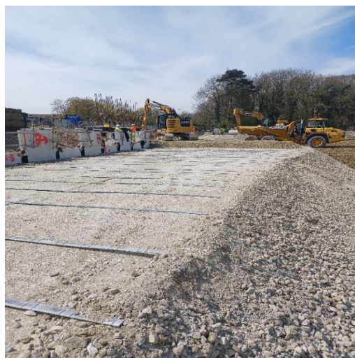
Wall panels installation in Section 1B North
