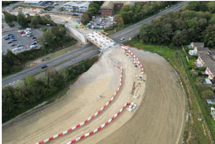
Image left shows view towards bridge and embankment.
