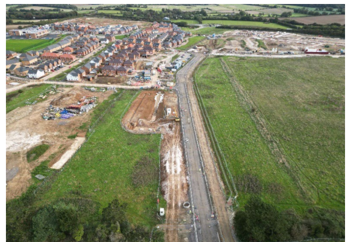
Image shows Drainage construction in Section 1a (towards Richmond Park)
