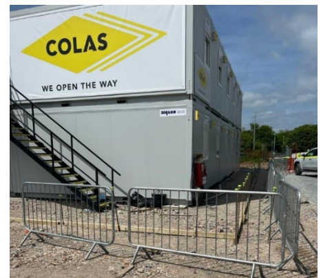
Figure 1 Colas Site Office
