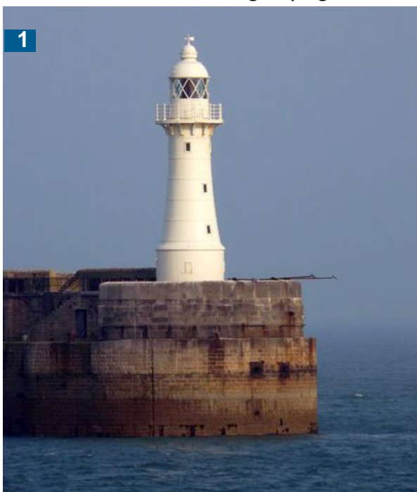
1. South Breakwater Lighthouse, Dover Harbour.
