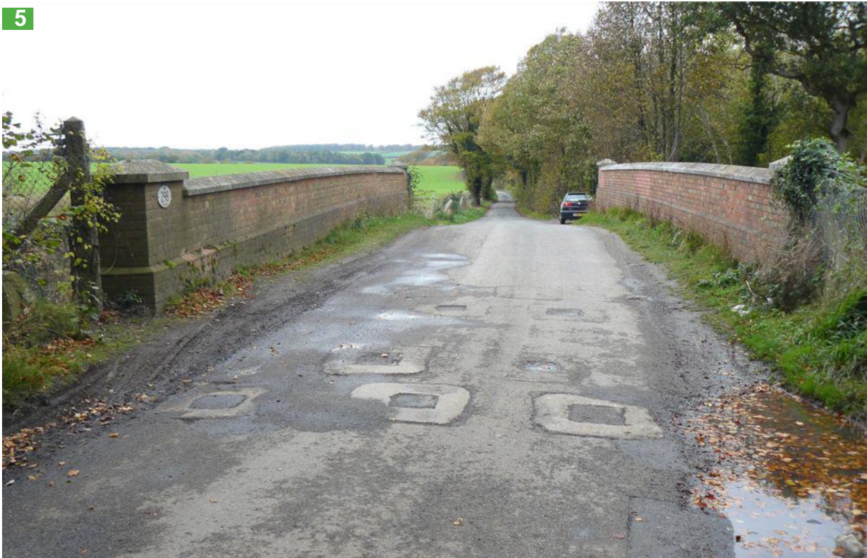
5. Scars in the road mark the position of a Second World War road-block on a bridge over the Dover to Canterbury railway line.
